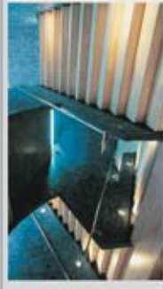
ERCO floor lights location: hallway to pool
